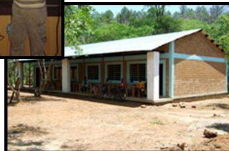
First completed classroom, Kapanda Community Day Secondary School
